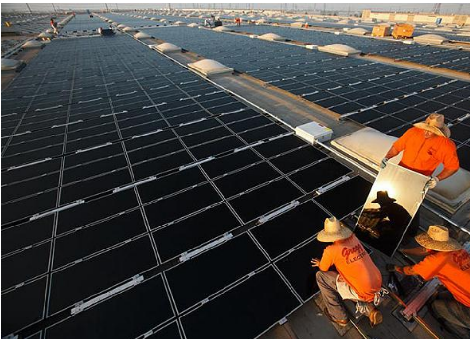
Turning unused space into a power source for 1,300 homes, Southern California Edison contractors cover a 14-acre warehouse roof near Los Angeles with some 33,000 lightweight photovoltaic (or PV) panels.
