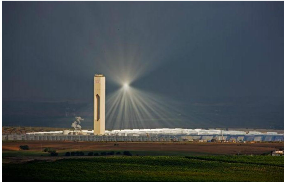
Above a scorched plain outside Seville, Spain, reflected sunlight reflects again off low clouds. Ordinarily the mirrors at Abengoa Solar's PS10 station beam searing, concentrated light to the top of the "power tower," heating a boiler that makes steam to drive a turbine. On overcast days, operators aim the mirrors skyward; sudden sun through clouds could heat the tower so quickly it could be destroyed.
